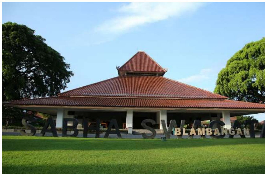
Sabha Blambangan Pavilion by the architect Adi Purnomo was revitalized as a public room, a discussion place, a book discussion location, and a new tourism place in Banyuwangi.
