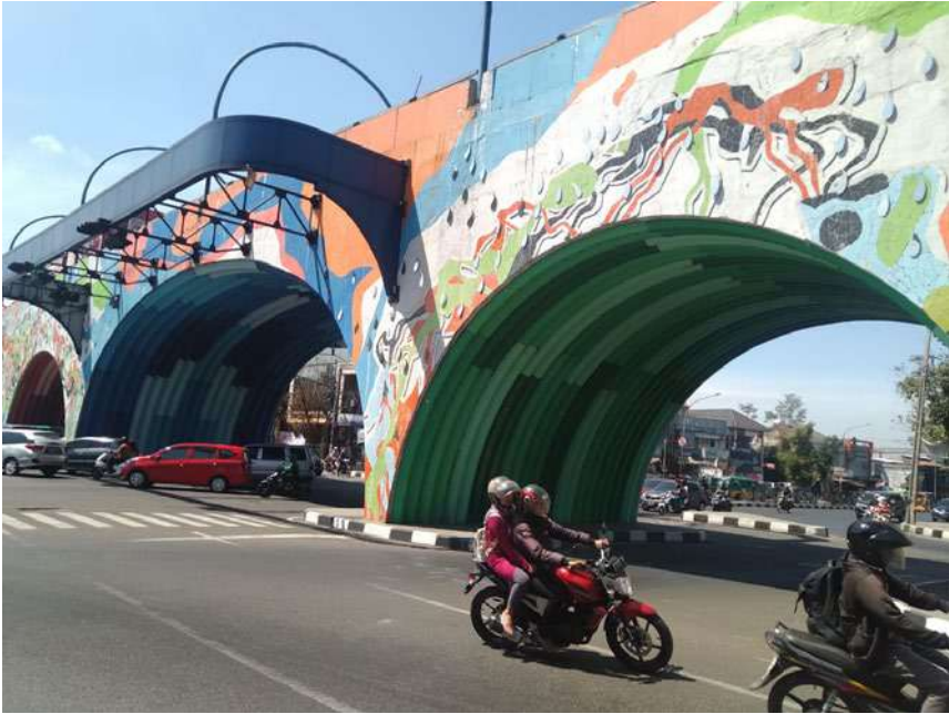
Antapani Bridge on Terusan Jakarta Street.
